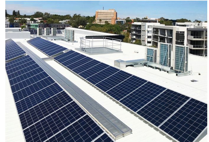
Phase I's 30kW photovoltaic system
